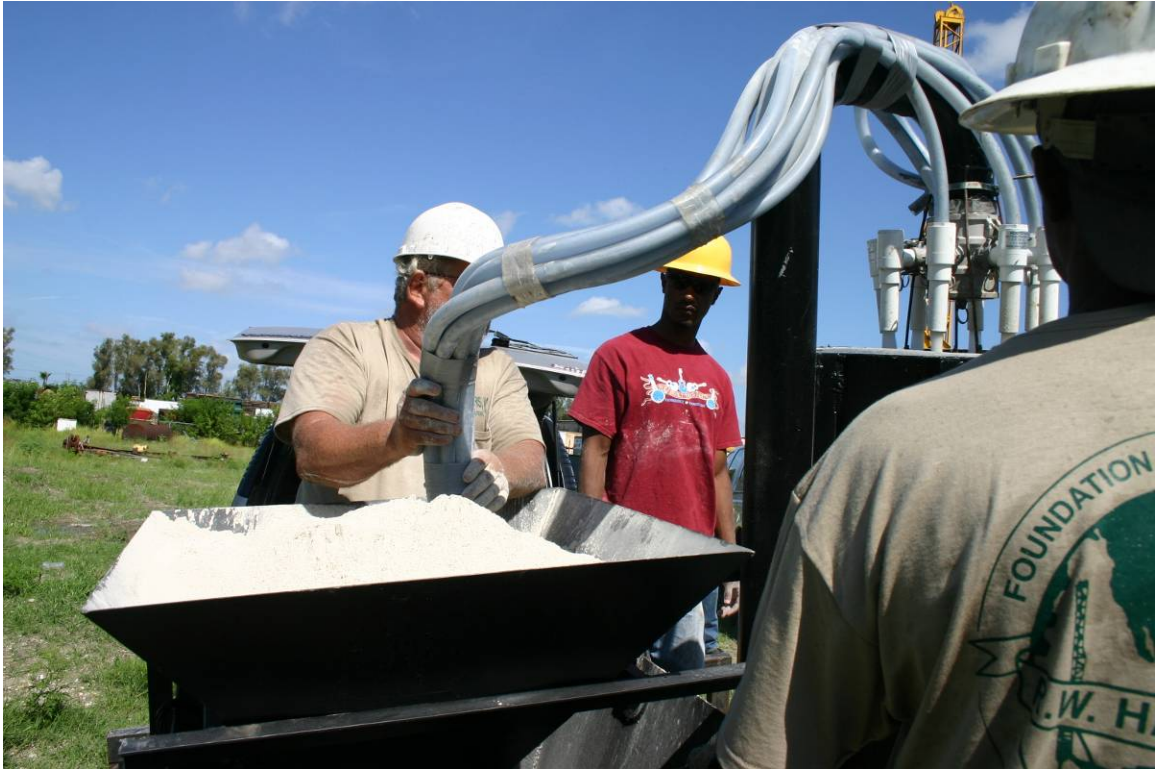
Figure 4.20. R.W. Harris personnel mixing drilling slurry with the multi-gang eductor system.
